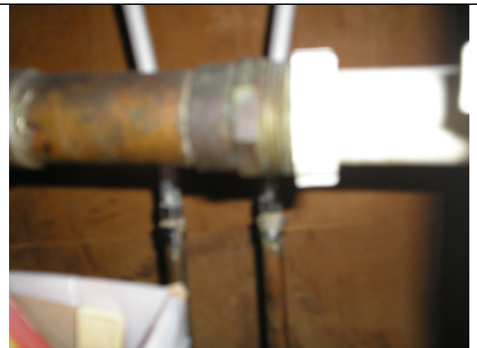
No water shut off valves under kitchen sink.
