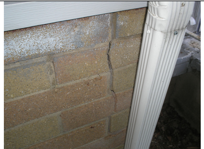
Crack in front fascia.
