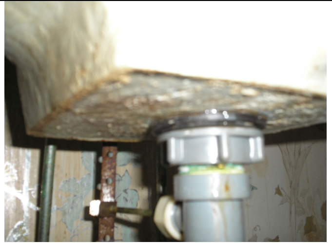
Leak under bath sink.
