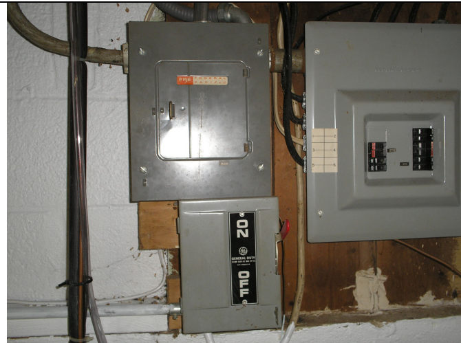
Disconnect in way of panel.
