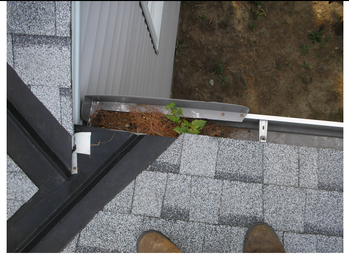
Debris in gutter.
