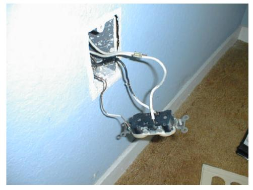
Figure 1 - Arcing Barrel Crimp Connection with Copper Wire
