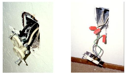
Figures 5 & 6 – Direct Wired Aluminum and Copper Pigtail with Old Style Wire Nuts
